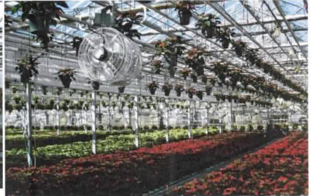
NRM's new retrofit motors use only 33 watts per motor, maintain the same airflow, yet operate much more quietly.
